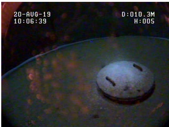
Floor centre access hatch appears intact
