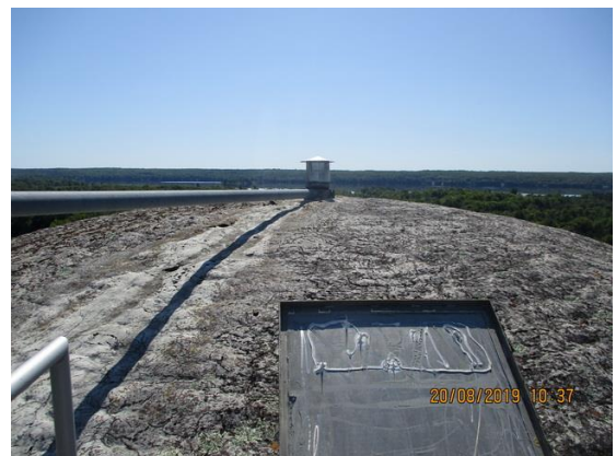
Looking at topside of domed roof and vent
