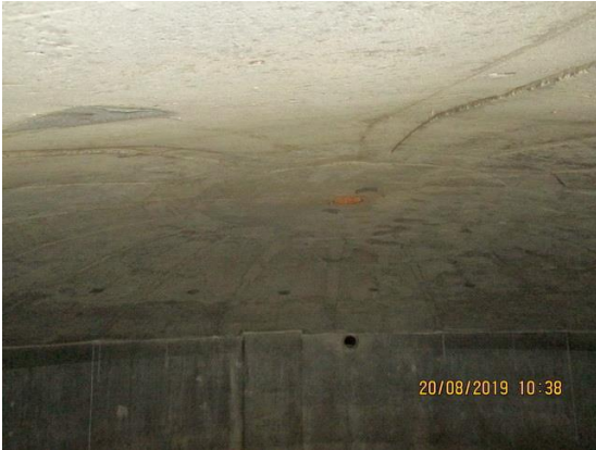
Underside of roof, vent and overflow opening
