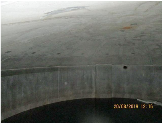
Looking across at tank underside and wall
