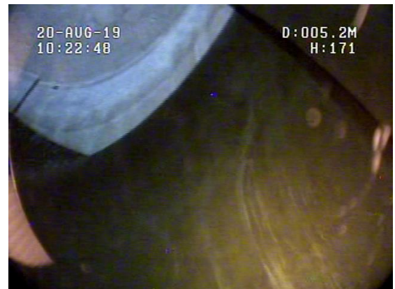
View looking up typical section of tank wall
