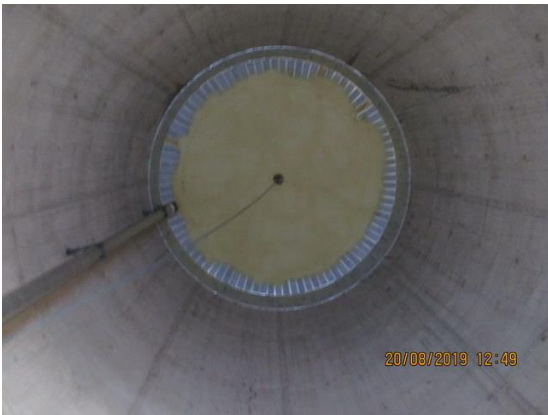
Underside of elevated tank viewed straight up
