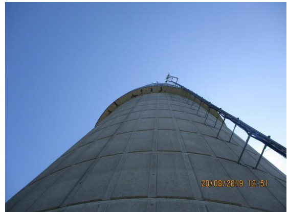
View up elevated tank support structure
