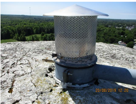
Roof vent appears intact and in good condition
