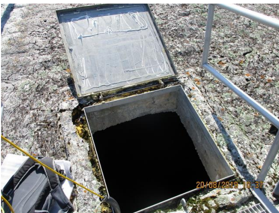
Roof hatch open during video survey
