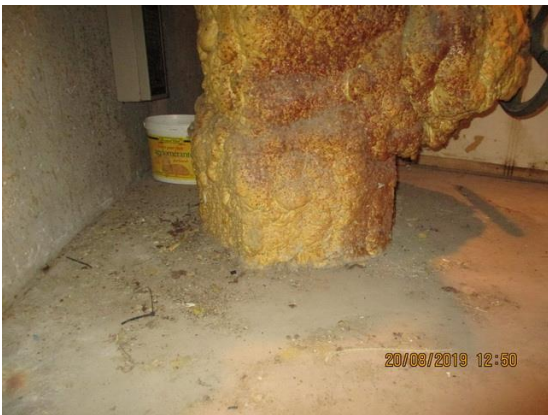
Floor-piping interface at grade level – no leaks seen
