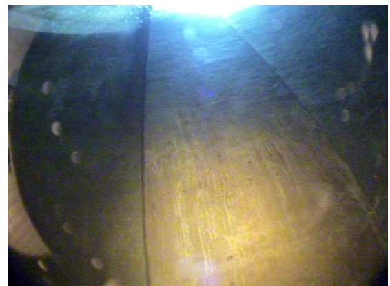
Underwater view up at vertical wall structure
