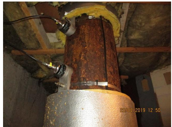
Bare section of outlet-inlet piping
