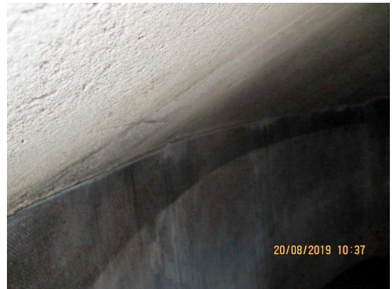
Look left from hatchway at roof-wall interface
