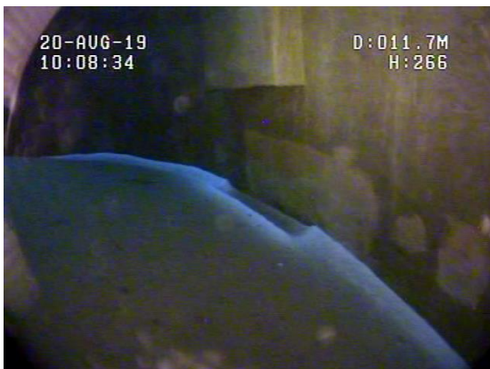
Outer floor sediment with white, powdery appearance
