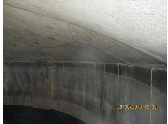
Look right from hatchway at roof-wall interface
