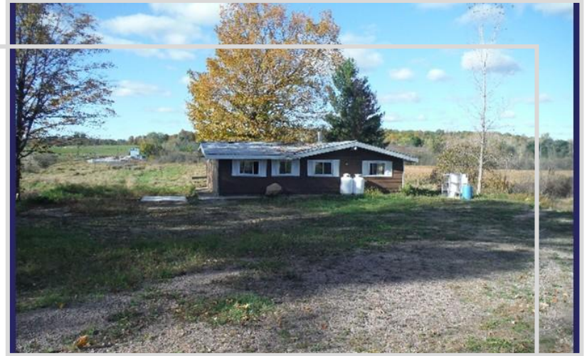
Non-Live Fire Training Structure
