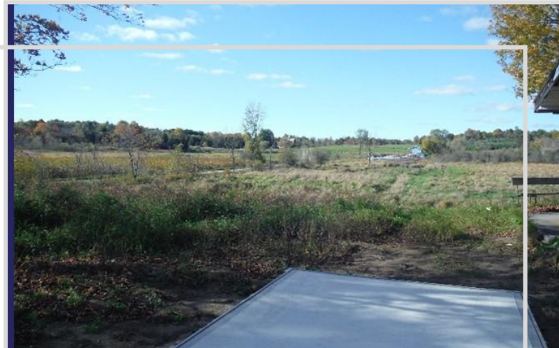
Live Fire Training Pad
